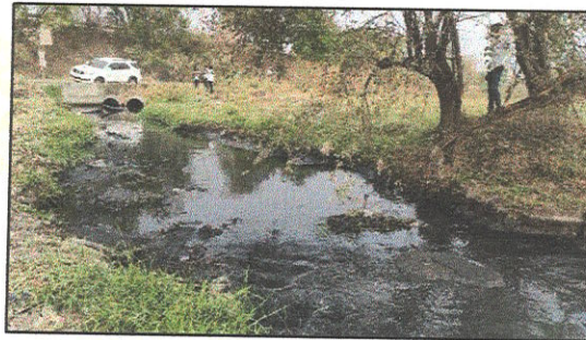
Figure 4 Sludge deposition in the nallah
