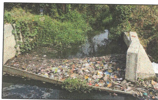
Figure 5 Solid waste dumping near the bridge
