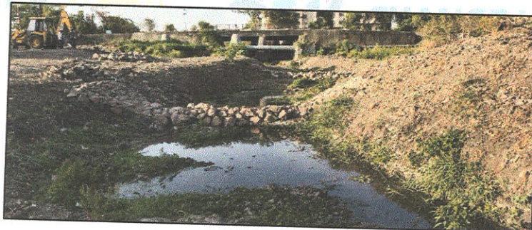
Figure 11. Instream structures near Symbiosis Gate 3 on the site
