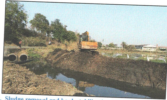
Figure 7. Sludge removal and bank stabilization near service road on the site
